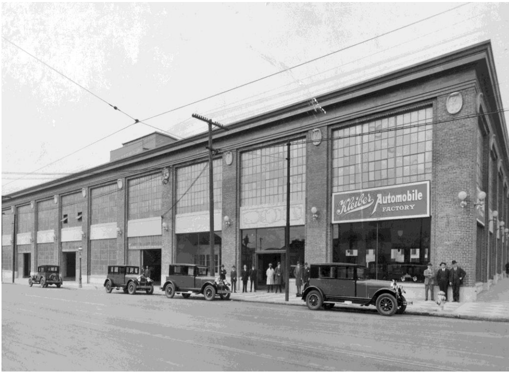
The new factory at 10 TH & Folsom. Notice the Kleiber cars parked outside and the showroom under Kleiber Automobile Factory sign
