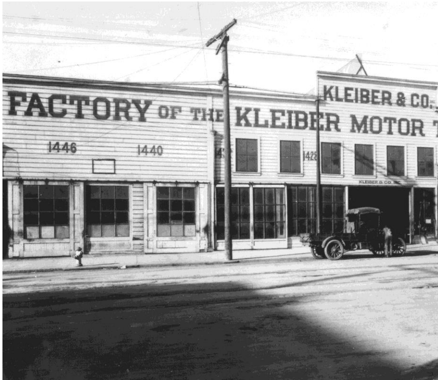
Old facilities at 10 th and Folsom San Francisco about 1918
